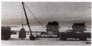
pulled. Although the lift can be pulled, it's much easier to control and maneuver if hooked to the front of the vehicle, says Empey. It folds down hydraulically for down-the-road transport at road speed.
