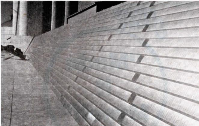
Galvanized steel walls bolt together without cutting or welding.
