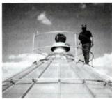
two semi-circular pieces create a rail about 8 ft. in dia. Simple mounting brackets and drill screws are provided for easy installation. A 2-screw hold-down strap screws into each rib on the roof. The rail, which sells for \$112, is made from 1-in. dia. galvanized tubing. One pair of rails weighs just 40 lbs. (Vince Steffen, Harvestall, 3 North Walnut Ave., New Hampton, Iowa 50659 ph 800 722-7544)
