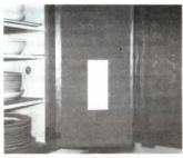
of the door and applied contact cement and then put on 1/4-in. thick cork board. I've fixed up two cupboard doors to hold recipes as well as the grocery list. (Nick Rogalski, Melville, Sask.)
