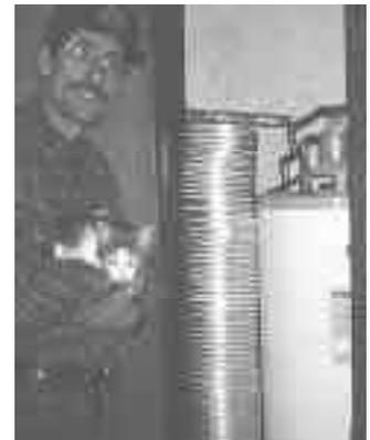
Space heater taps into hot water line and runs through stove pipe mounted on side of water heater.
