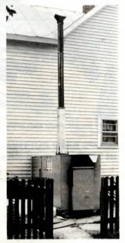
sits outside the home and only the hot and cold air ducts and thermostat wires enter the living space," says Cauffman, noting that Sure Flame, Inc., is in the process of finishing testing on final prototypes. Both forced air and hot water 200,000 btu models will be available for a price of around \$2,000.
