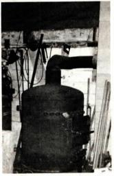
near the top of the stove. Hot air from the firebox rises through the pipes on its way out the chimney. A 110-volt fan, which attaches to the back of the stove, blows air through the pipes and into the shop.
