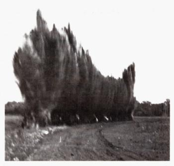
Two-man crews can ditch up to about 1,000 ft. per day with dynamite. Explosion spreads dirt over wide area, eliminating ridges along ditch.
