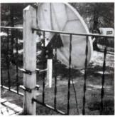
The dish rests inside a piece of pipe held by two large bolts that run to a pair of clampon brackets on the deck post. This setup gets the dish up off the ground, makes it easy to make adjustments, and puts it above the level of trees and shrubs.
