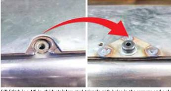
Sill Stitch is a 1/8-in. thick stainless-steel triangle with holes in the corners and a slot in the center. The corners are welded to the top side of the header plate, and a new bolt and washer are installed.
