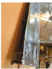
Metal is spaced 4 in. from wood walls and with a 5-in. bottom gap to circulate heat away from walls.
