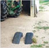
Fritz Groszkruger, Dumont, Iowa: "The sliding doors on my pole barn used to be held in the center by a buried post with a welded piece that fit between the rails. It didn't hold up, so I came up with the idea of using a pair of buried truck tires, spaced so the doors slide between them. Works much better.
