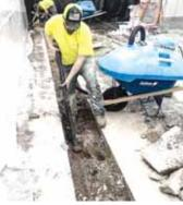
Roll-N-Vac is designed to vacuum directly into a wheelbarrow.
