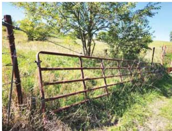
**Gates held in place by steel cable anchored to top bar of gate and steel pipe.**
