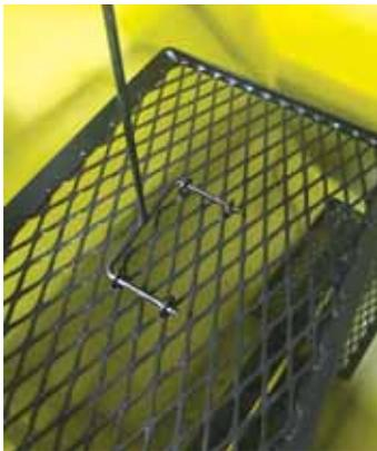
Van Well planter grate shown with lift bar to clear debris that would've gone into the planter.
