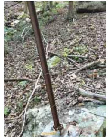
Using a cordless 20-volt DeWalt hammer drill, he drilled two holes through the plate into the rock for two concrete wedge anchors to bolt to.
