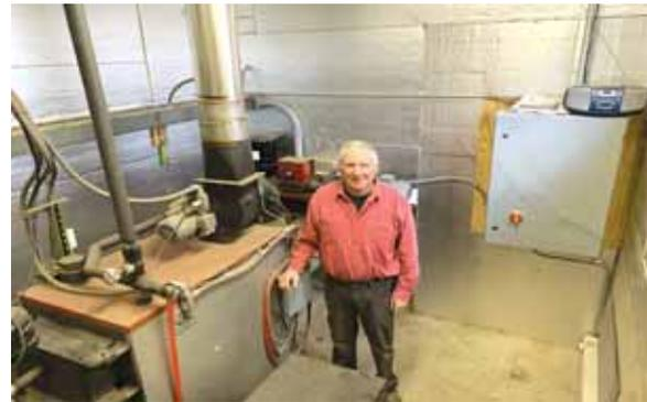
Kramer fitted a boiler with a chopper and feeder system to use loose hay.
