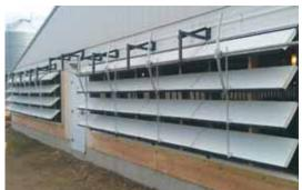
Their unique rack and pinion drives are fitted with limit switches providing the exact torque and speed to properly operate the shutters.
