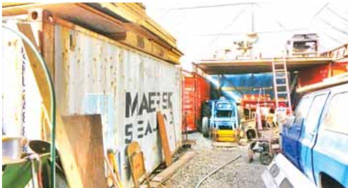
Stover's workshop was made using four shipping containers with a crushed rock floor and hoop house roof.
