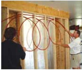
PEX tubing is looped through holes drilled in wall studs.
