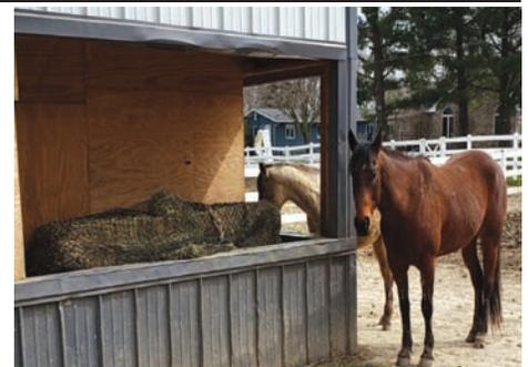
Two-sided feeding station was built by cutting out two 6-ft. high openings in the corner of horse barn.
