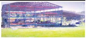
Karkau got 350 8-ft. and 12-ft. pallet rack cross members from an old warehouse for \$400. As a bonus, the price included 100 sheets of 3/4 and 1/2-in. plywood, which he used for divider walls and adding a second floor to his building.
