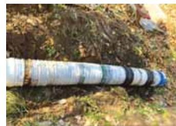
**5-gal. buckets with the bottoms removed are stacked together to create a heavy-duty pipe.**
