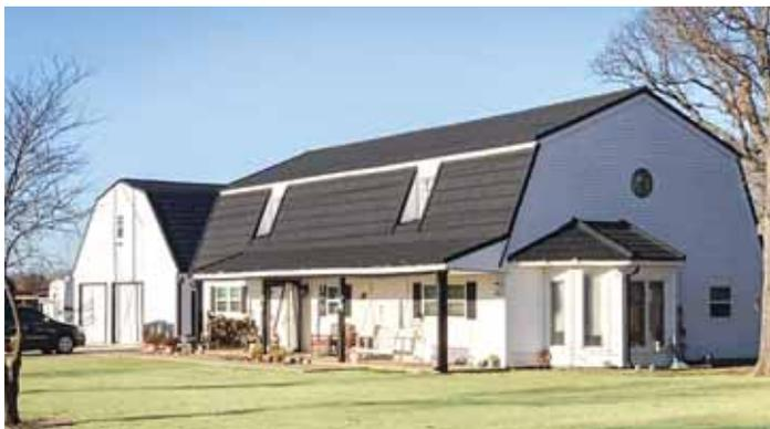
Metal roof panels of 26-ga. stone coated steel measuring 3 ft. by 20 in. feature an acrylic base coat and have the same stone granules used in asphalt shingles.
