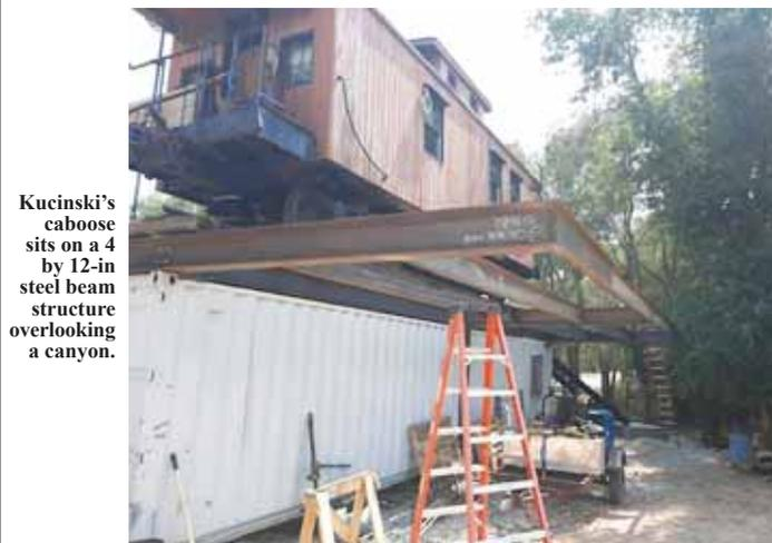
**Kucinski's caboose sits on a 4 by 12-in steel beam structure overlooking a canyon.**
