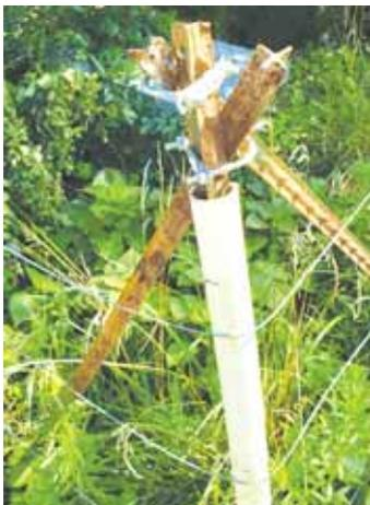
**U-Bolts are used to attach brace posts at an angle making a secure corner post.**
