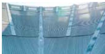
Perforated louvers make up the second floor forcing air into the grain.
