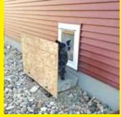
I used mostly scrap material to build a cozy 3-ft. high, 6 by 4-ft. dog house in our garage. It keeps our dog warm in cold weather. The garage wall forms one side of the dog house, and a commercial "doggie door", consisting of 2 clear plastic flaps, leads outside the wall to a step and a plywood windbreak. The doggie door came with an extra panel that can be slid on outside the door to lock it up.
