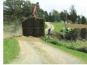
Old bridge deck was removed with a big backhoe and placed temporarily upstream to carry light traffic during construction.
