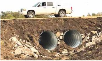
A contractor replaced the 70-year-old bridge on Gogerty's farm road with two 28-ft. long corrugated metal drainage pipes.
