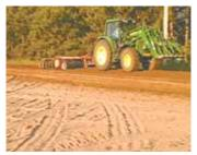
Farm equipment is all that is needed to prepare the soil and mix the solution. An industrial roller or packer will do the best job compacting. Discs and rototillers may also be used to mix the soil. After the correct grade is achieved, compacting is
