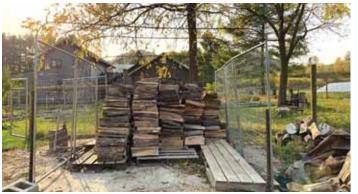
Ruen used 6-ft. tall panels to create two 15-ft. long walls. Four 20-ft. concrete reinforcing rods, bent into U-shapes, slip into panels' open uprights to support tarp.
