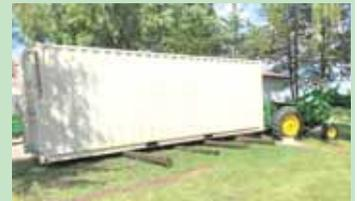
To move the container without gouging the grass, Rinke lifted it with the 3-pt. jig and set it on round wooden fence posts. "It rolled along real well and I was able to maneuver it in place on the footings very easily with the jig," Rinke says. "If money was no object it certainly would've been easier to have a cement pumper truck and a lift crane do the work, but I enjoy the challenge of building things that get a job done efficiently and economically."
