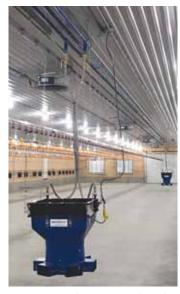
Hot water supplied by an exterior boiler is piped to individual heat exchange units inside poultry and swine buildings.
