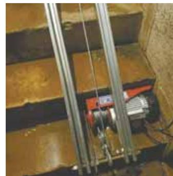
**Electric hoist fits under tracks on bottom basement step.**
