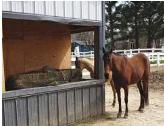
Two-sided feeding station was built by cutting out two 6-ft. high openings in the corner of horse barn.
