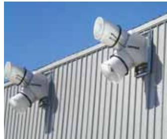
A turbine fan forces fresh air into a system of corrugated tubing encased inside a 20-ft. ventilation duct.
