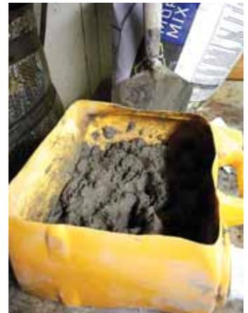
Big laundry detergent jug has one side cut out. Lakatos holds onto jug handle while stirring the concrete.
