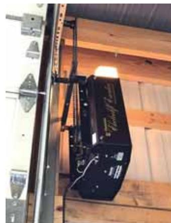
Larry Wood gained more overhead room in his shed by converting a standard overhead garage door opener to a side-mounted one.
