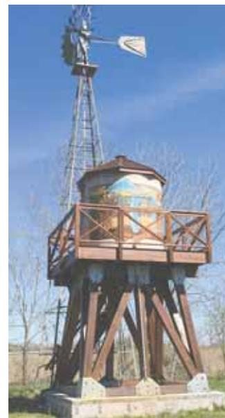
Paul Behrends built this 3,000-gal. wooden water tank for a customer who uses it to drip irrigate an orchard. Tank is filled by 50-ft. windmill in background.
