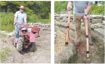
Ruen used plastic tubing and 2 yardsticks to make a water level for maintaining grade, while using a rototiller to dig a 190-ft. long drainage ditch around his house.
