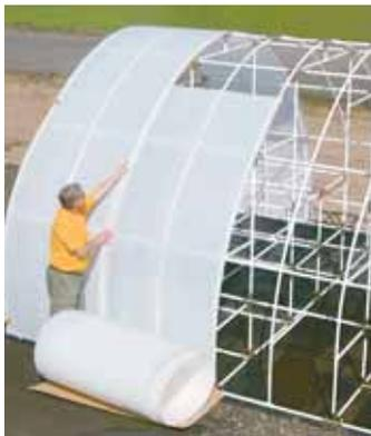
Flexible, twin-wall Solexx is a high-density polyethylene that provides a permanent greenhouse cover in snow and high wind areas. It comes in ready-to-install rolls.
