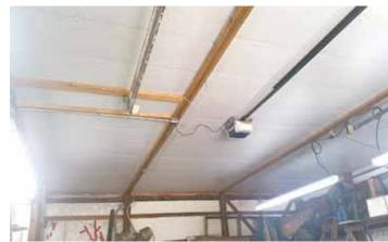
Brauer installed 2 by 2's at the bottom of the trusses in his shop and laid in garage door panels, then added  $3\ 1/2$  in. of insulation on top that's covered with Tyvek.
