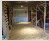
They covered the crib with used steel siding, built a pair of large sliding doors, and painted the building red with white trim. They also filled the alley with gravel.
