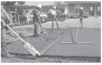
build drive-over curb and gutters and valley pans in a single pass.
