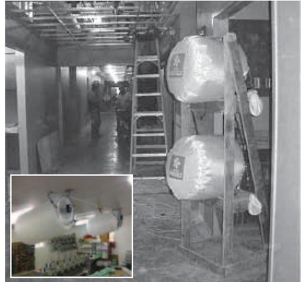
**Demo Air Net filter/net fits over discharge end of a fan and is secured with a bungee cord. It can be used for everything from workshops to barns and homes.**
