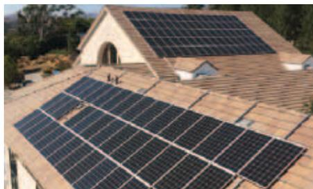
No roof penetration (SolarPod™ Crown) solar system. Installs on all roof materials - shingle, metal, tile and wood.
