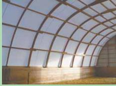
Silver Stream makes hoop barns with either steel or wood hoops. The advantage of wood is that it's easier to insulate and it can be tinned over at any time, if desired.
