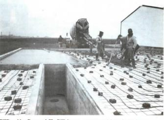
BillBroaddus, Raymond, III.: Bill's happy with the in-floor heat system he installed in his 54 by 54-ft. farm shop. He ran pipes under the floor of the shop and pumps hot water through them with a gas-fired boiler. To install the system, he worked closely with the manufacturer of the equipment he bought - Heat Way, 3131 West Chestnut, Springfield, Missouri.
