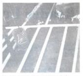
We laid hot air pipes underneath the concrete floor of a new heifer-dry cow barn we built in 1989. We used plastic sewer pipe to carry warm air from the milker pump exhaust to the floor of the dry cow barn. It keeps the floor under the alleyway and maternity pens thawed in cold weather. The cows are not locked in the barn - they're free to come in to eat and drink and then go back outside if they wish.
