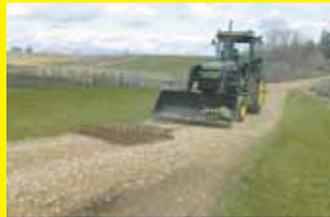
A double bed-size spring puts an excellent finish on newly spread crushed rock along our driveway. If needed, you can put concrete blocks on top for added weight on initial trips.
