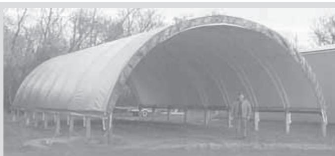
Grant Nelson bought and constructed this 30 by 80-ft. hoop-type building from Silver Stream Shelters. He put it up in about seven hours.
