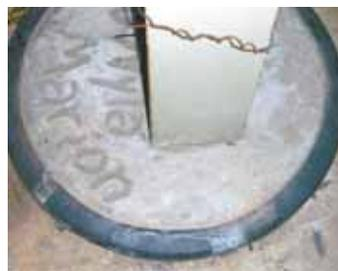
Vertical beam sets inside 6-ft. deep, 18-in. dia. hole lined by a ribbed poly culvert and filled with 2 ft. of concrete.
