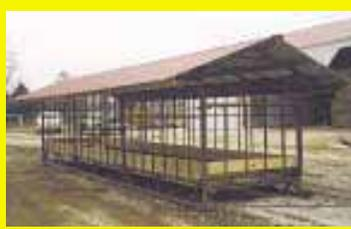
ing while a wooden floor is built of treated 2 by 6's or 2 by 10's. You can easily move it to new locations around the farm with bottom runners, which are constructed of 4-in. dia. pipe turned up on each end so you can pull or push the feeder with a 4-WD pickup.
