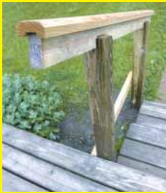
Here's a simple handrail for a 2 by 4 stairway railing. It fits over another 2 by 4 set on edge. Just cut a dado that's sized to fit over the side of the 2 by 4 and then bevel the top edges. Gives a finished look to the railing and a better grip. **(Dillon Phillips, Indianola, Iowa)**
